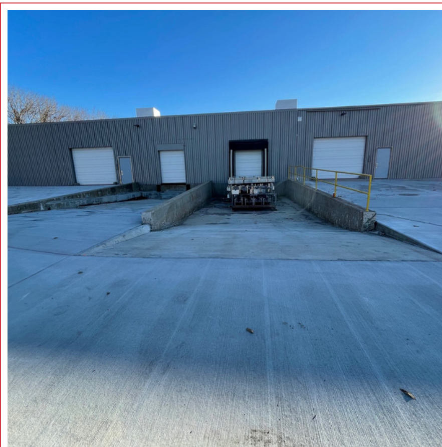
Building A — Rear Truck Court & Loading
