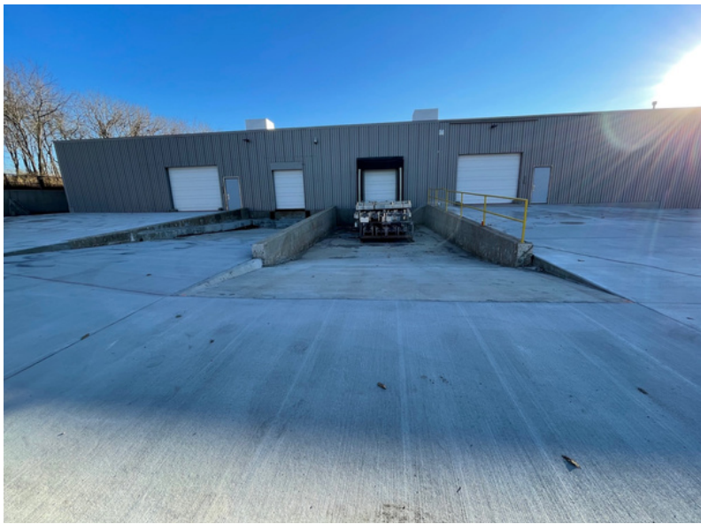
Rear Truck Court — Dock & Drive-In Loading
