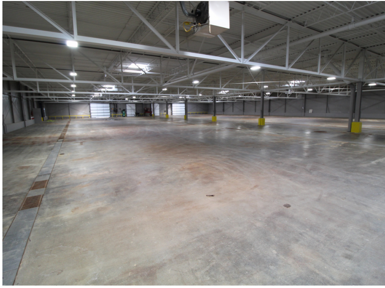
Warehouse — 168' x 129'6" Clear-Span Bay
