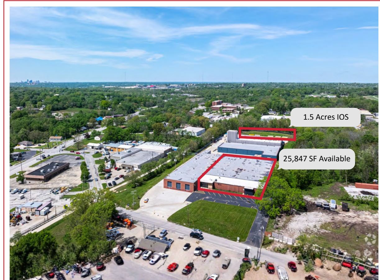
Building A — Front Elevation on E 56th Street
