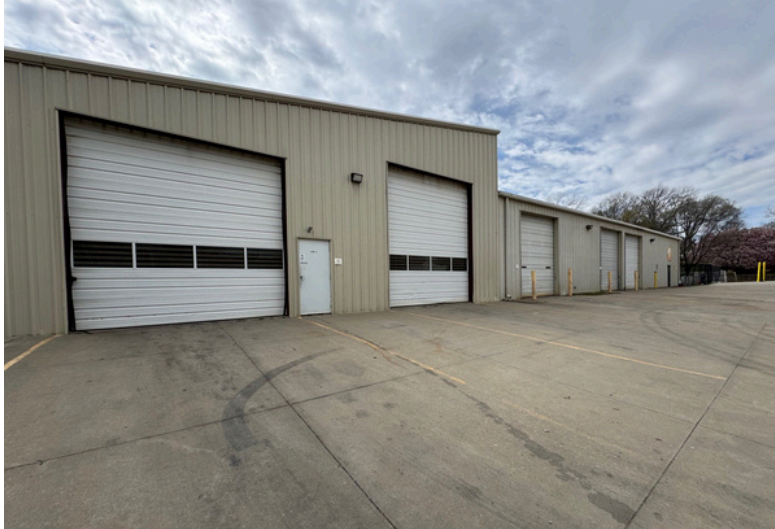
Front of Building
